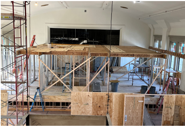
Face to Face is growing! Construction is underway to transform part of our gym into much needed office and meeting space. It will create private, welcoming areas where guests can receive support with dignity and respect.
